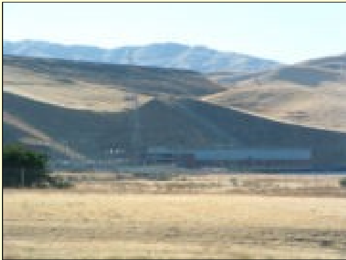
San Luis Dam near Los Bonos, California – an Embankment Dam
