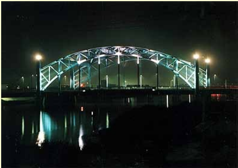
Meiwa Bridge, Edogawa-Ku, Tokyo
