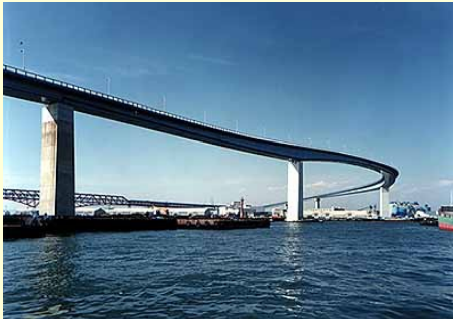
Namihaya Bridge, Osaka, Japan
